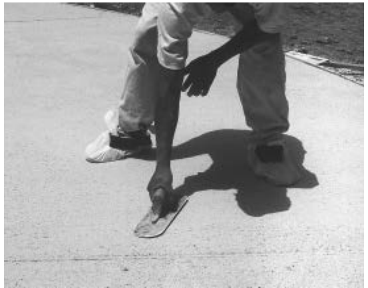
Above: Soft plastic bags allow the finisher to apply the final pass without leaving foot prints.
