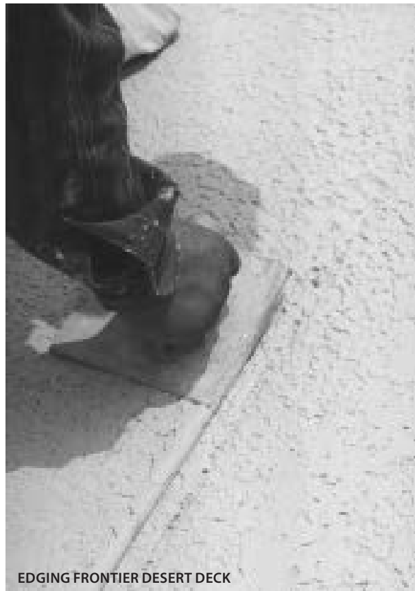
Above: Soft plastic bags allow the finisher to apply the final pass without leaving foot prints.
