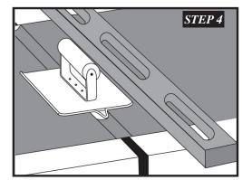
**Step 4.** Tool the joints at the appropriate time using the lay-out marks as a guide.
