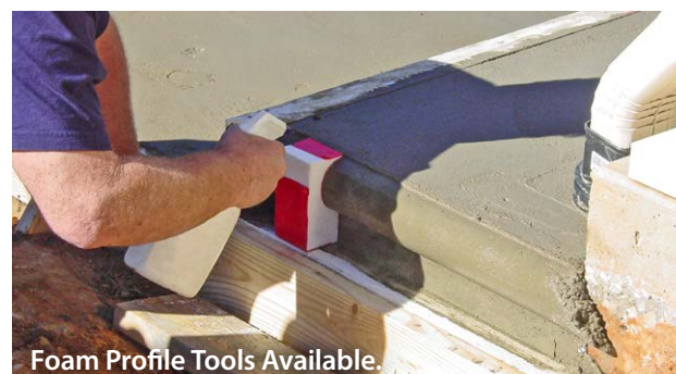
Use spray adhesive or nails to attach.
